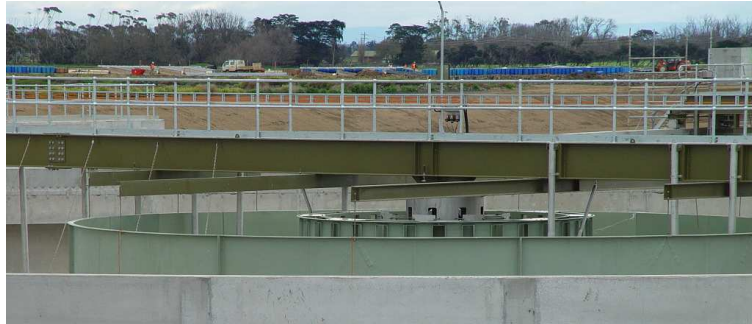
Figure 7 Prototype of Modified Central Inlet Structure
